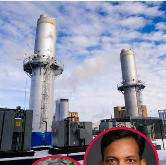
The central utilities plant is the industrial heart of a university campus, distributing the electricity, steam, hot water and chilled water needed to run air conditioning systems and research facilities to multiple buildings.
