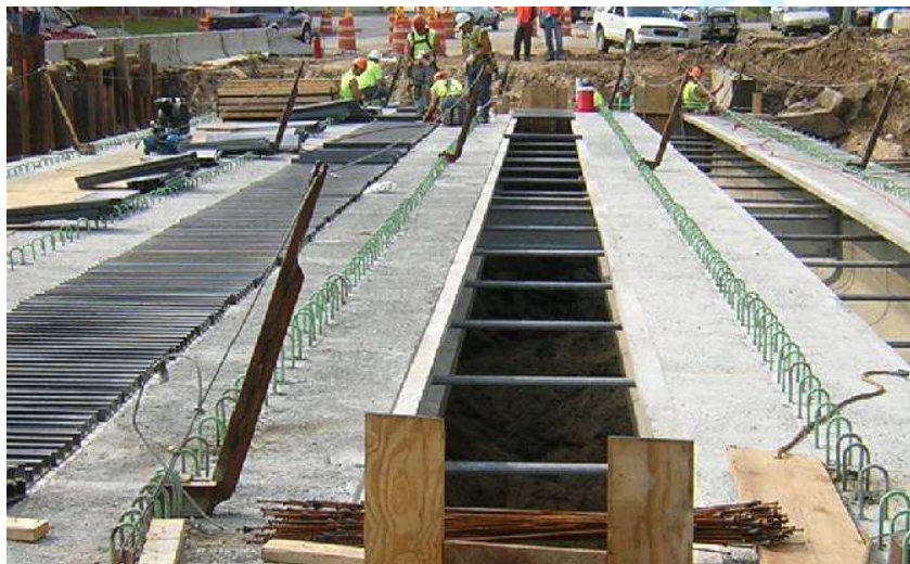
7 8 Fig. 3–Construction of a pilot bridge with a reinforcement-free bridge deck.
